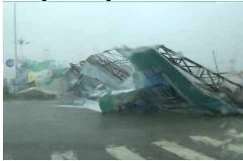
Fig.17 Collapse of advertising board
