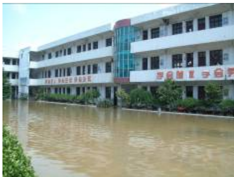
Fig.19 Flood at an elementary school
