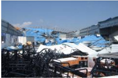
Fig.15 Damage to work shed
