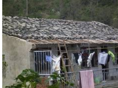
Fig.10 Stone placed in roof to protect roof
