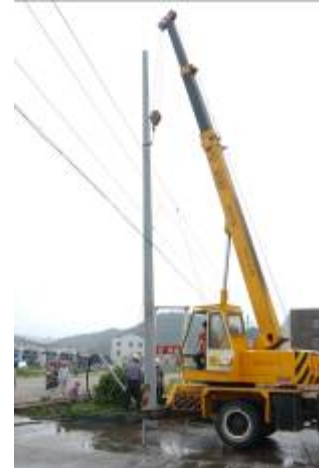
Fig.20 Repairing electricity pole
