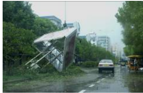
Fig.16 Collapse of advertising board
