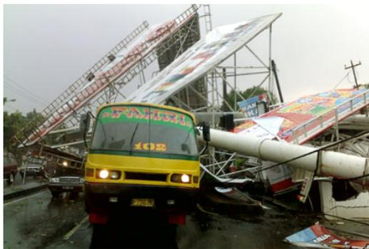
**Figure 7. Damage due to bill board overturning**
