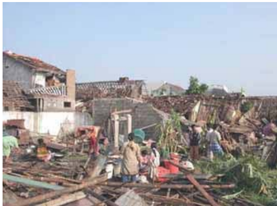
Figure 5. Damages in slum area
