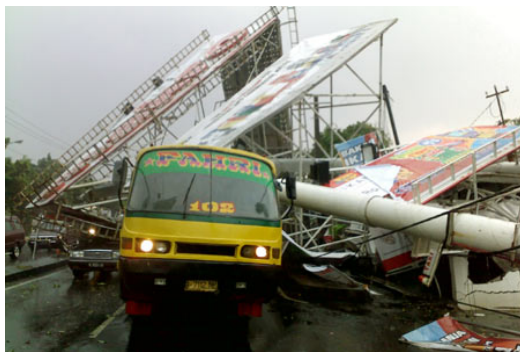
Figure 7. Damage due to bill board overturning
