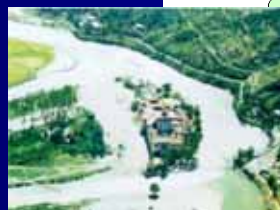
Damaged area in Punaka city
