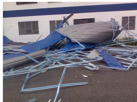
Figure 1b – Steel Truss failure
