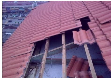
Figure 4b: Damage Roof Tile
