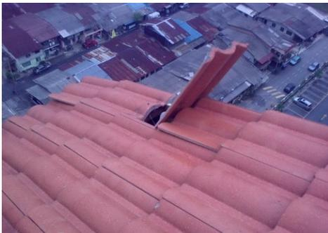
Figure 4a: Uplift Roof Tile
