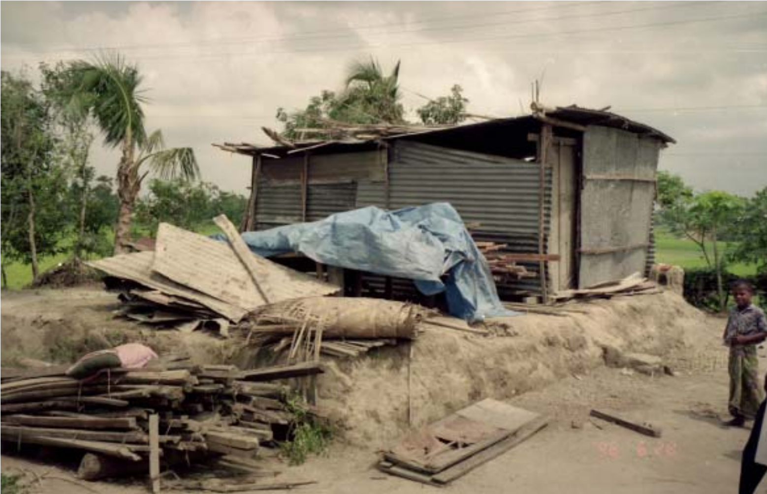
Fig.10 Tin roof and wall house
