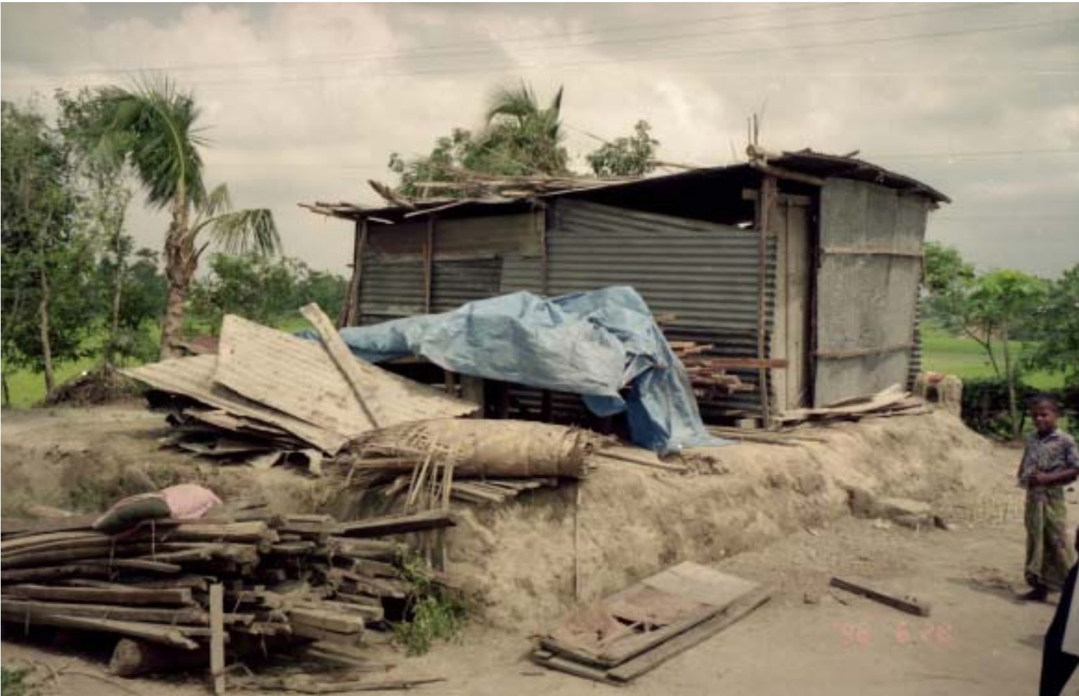
Fig.10 Tin roof and wall house
